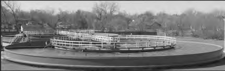
Wastewater Treatment Solutions
