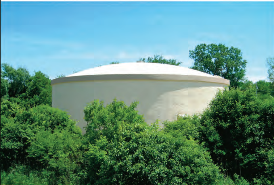
1.0 MG Natgun water tank for the Village of Posen, IL. Engineering by Robinson Engineering, Ltd., South Holland, IL.
